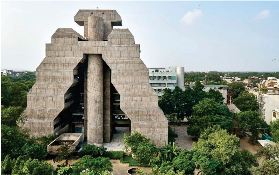
NCDC HQ Building exemplifies a spirit of cooperation
